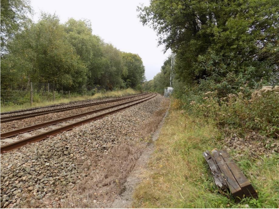
Figure 2-4.3: Railway in the Up direction from the Down side
