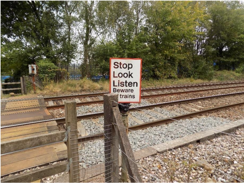
Figure 2-8.2.2: Signage on Down side
