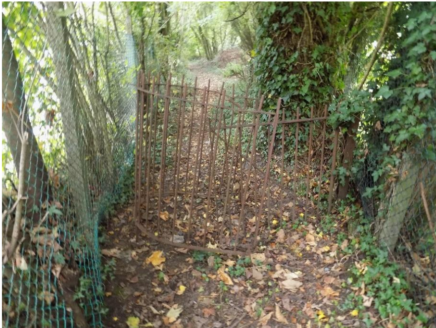
Figure 2-3.6: Up side approach to Wernddu Footpath Level Crossing
